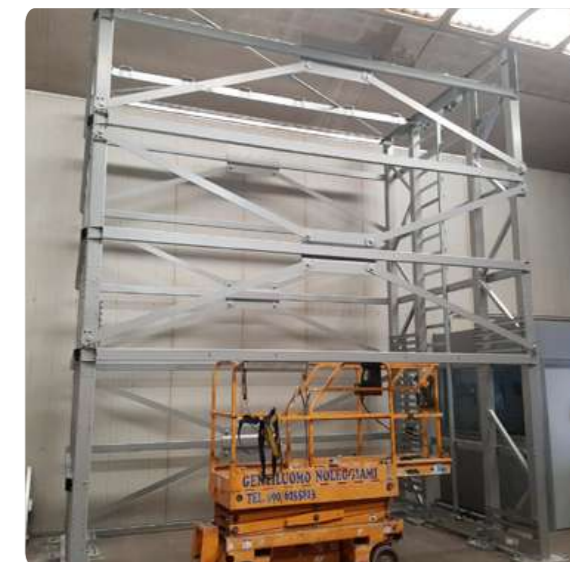
REINFORCED EARTHQUAKE-RESISTANT STRUCTURE
